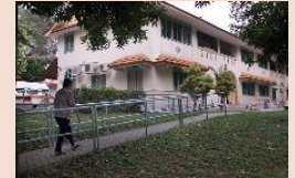
Changi 120 beds Retrofitted
